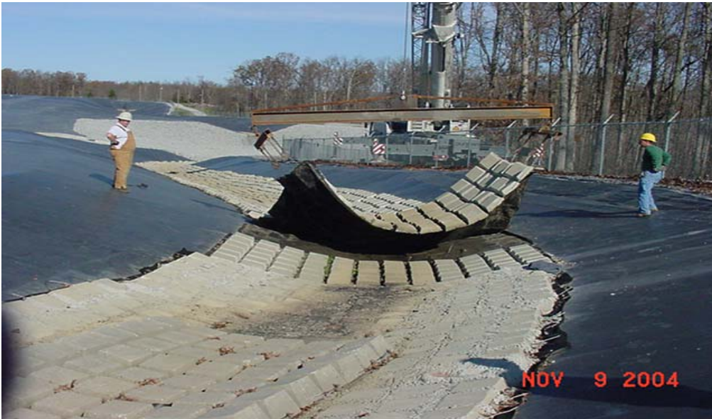
Photo 2 AB mats in Southeast channel being lifted for realignment
