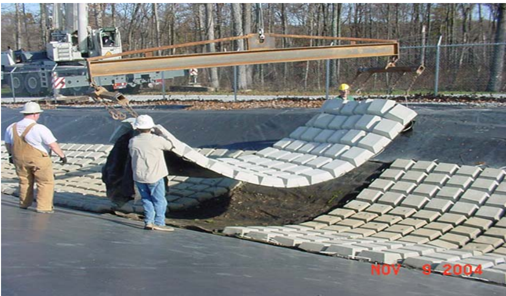
Photo 3 New cc45 mat being installed
