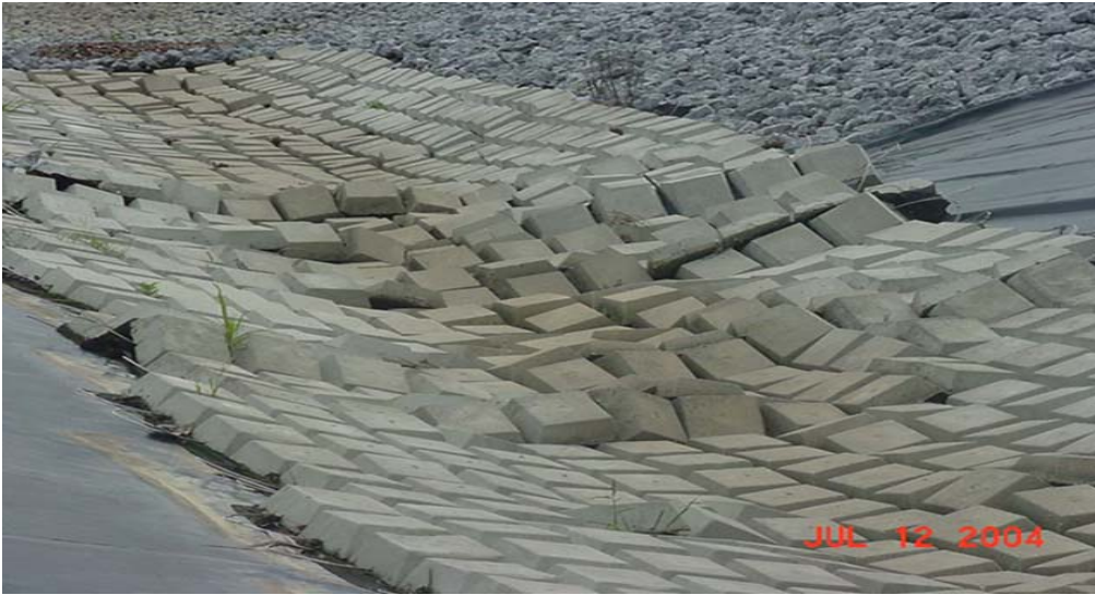
Photo 1 AB mats in South Channel following major rain event.
